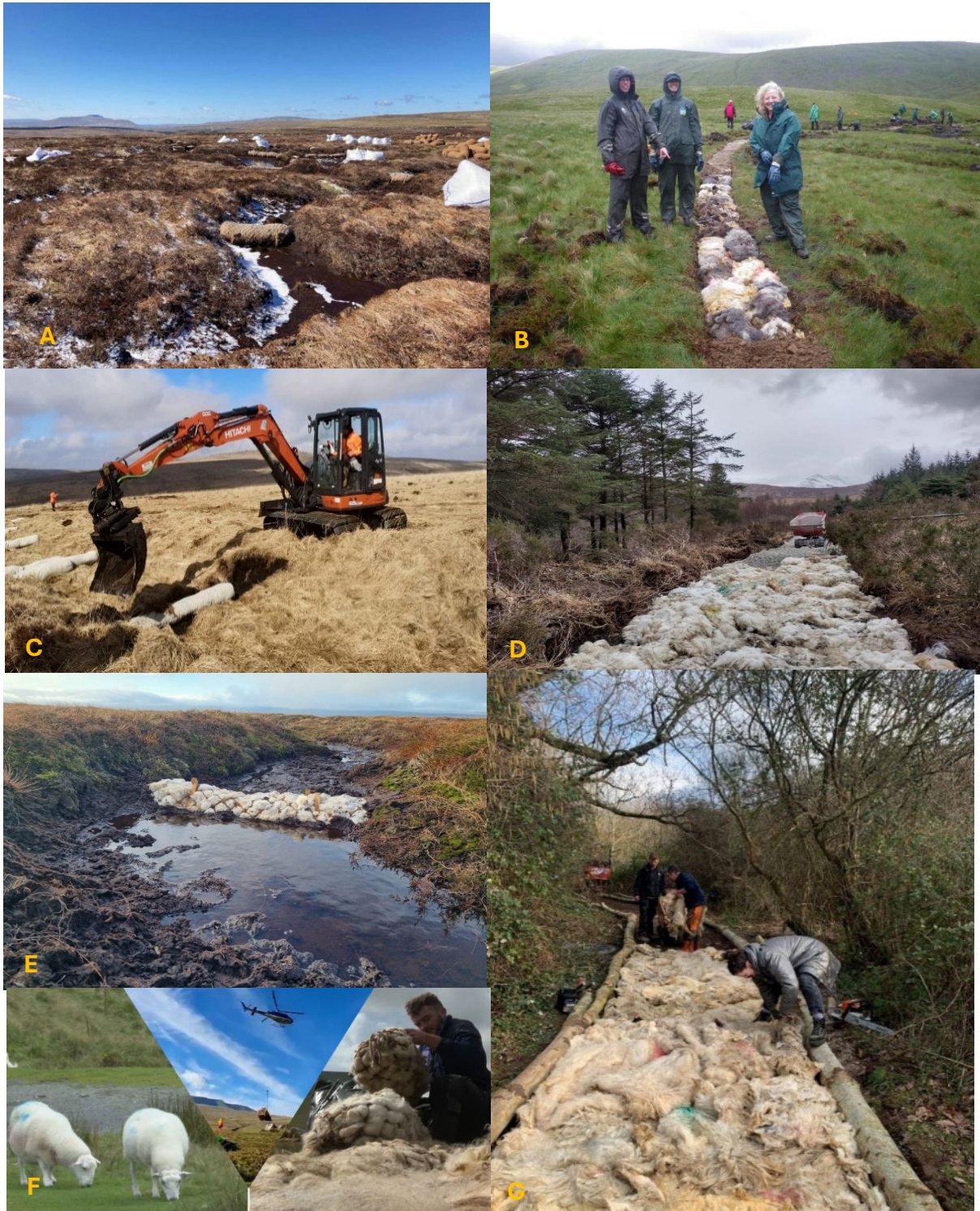
Figure 8 A: Wool-filled felt tubes installed on Dartmoor's peatland to slow water flow and support bog plant growth. E: Sheep's wool used in the North Pennines AONB to reduce erosion and retain carbon in peatland restoration 8 F: Wool blankets placed in Welsh peatlands to slow water flow and protect carbon-rich soils, aiding climate resilience C: 9 Wool logs placed across Fleet Moss in the Yorkshire Dales to combat erosion and support peatland restoration. D: Sheep wool used on the Isle of Skye to create a durable, eco-friendly path that protects peat and improves drainage. B: Volunteers with Fix the Fells use sheep fleece to reinforce paths, control erosion, and protect peat in the Lake District G: 10 Welsh wool used to create sustainable footpaths, reducing plastic reliance and promoting eco-friendly infrastructure.
